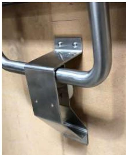
3. Attach wall bracket by sliding the open end over the support bar whilst the seat is in the vertical upright position.
