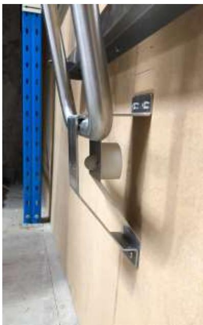
5. Fasten using mounting holes provided at the bottom of the wall bracket.
